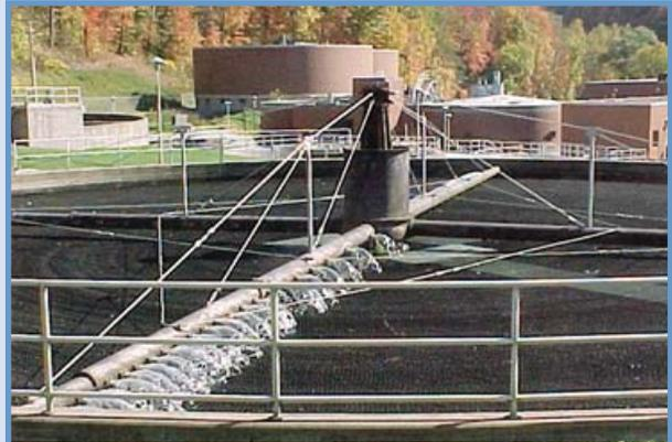
Franklin Township (Murrysville, PA) Wastewater Treatment Plant. Foreground is media trickling filter, background is nitrification towers (left) and sludge digesters (right).
